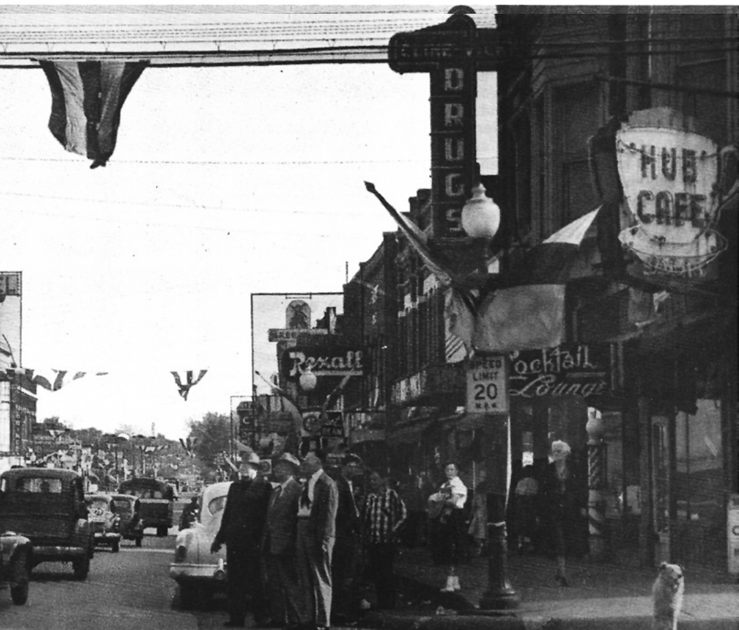
Illinois Avenue looking south from Main Street, note two-way traffic.
